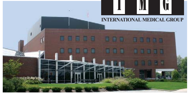
IMG World Headquarters, Indianapolis, Indiana
