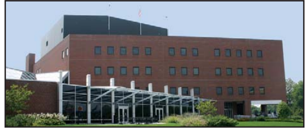
IMG World Headquarters, Indianapolis, Indiana
